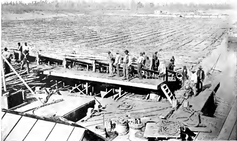
FASCINE MAT UNDER CONSTRUCTION.
